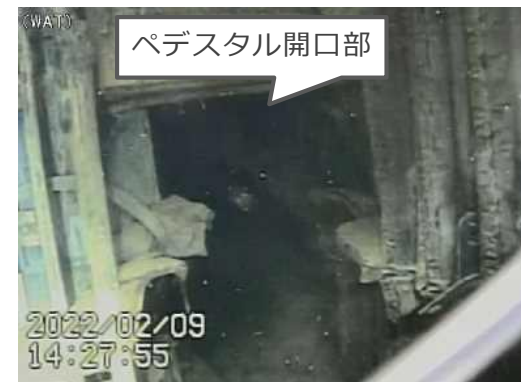
ペDESTAL開口部俯瞰
