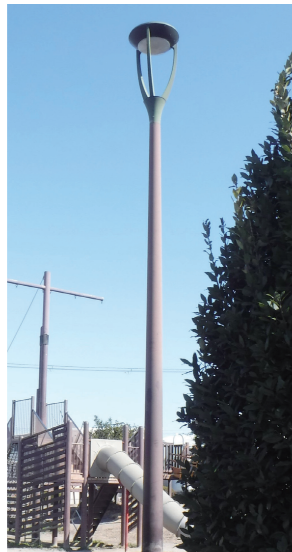
LED 化工事前
