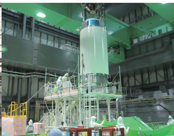
Removing fuel from the spent fuel pool of Unit 4
