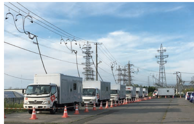
High-voltage generator trucks dispatched to the disaster area in Hokkaido (September 2018)
