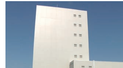
May 2015 Completion of a large rest area The facility includes a cafeteria and a convenience store (March 2016)
