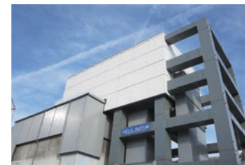
December 2014 Completion of fuel removal from Unit 4 Work to remove the fuel from the spent fuel pool and transfer it to the common pool began in November 2013. As of December 2014, all 1,533 fuel assemblies had been moved.
