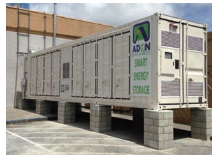
Installation of storage batteries in Hawaii (Oahu) (TEPCO Ventures)
