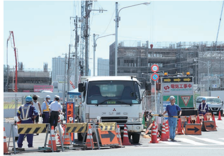
Construction site of athlete village (Koto District, Tokyo)
