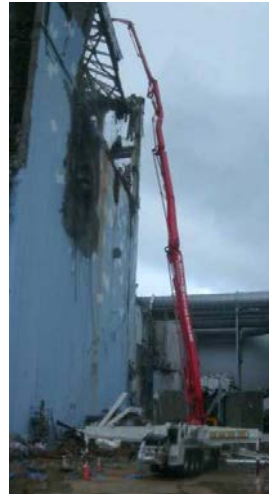
Concrete pump vehicle/Germany
