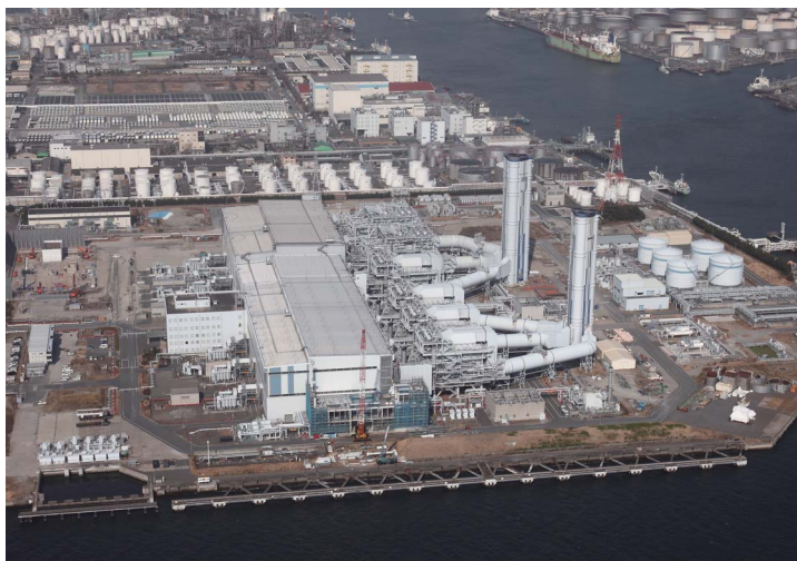
The Kawasaki Thermal Power Station Group 2 upgraded its second power generation turbine with the introduction of the MACC II,* bringing it online * More Advanced Combined Cycle II
