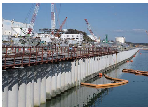
Impermeable walls on the shoreline were completely sealed in October 2015
