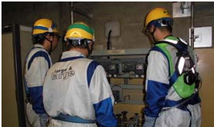
Onsite checks by TEPCO employee (on the right)
