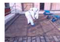
Concrete removed from top of office building
