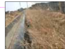
Before conduit covering
