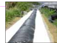
After conduit covering
