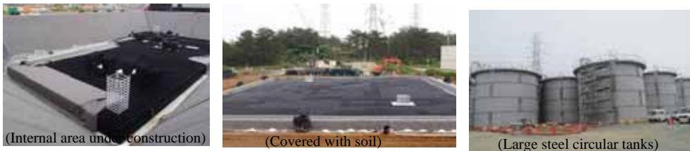
< Status of installation of underground storage water tanks >
