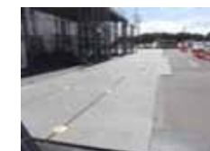
Commuter bus stop (after shielding)
