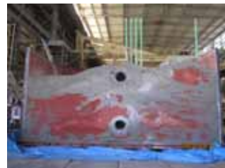
Layering of water stopping material after injection
