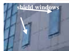
Main office building window shielding
