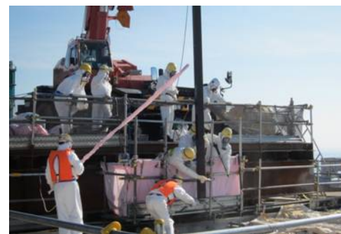
Fig. 5 Removal of fresh fuel from Unit 4 Spent Fuel Pool
