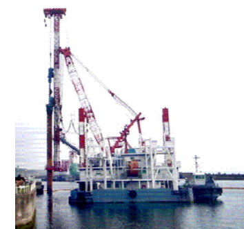
Fig.2 Impermeable wall advance excavation work
