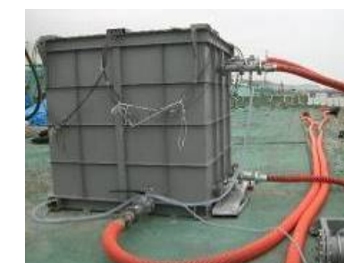
Fig.3 Operation of seawater circulation purification apparatus
