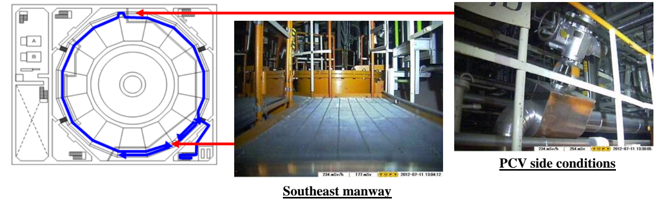
Fig. 6 Unit 3 Torus Room investigation
