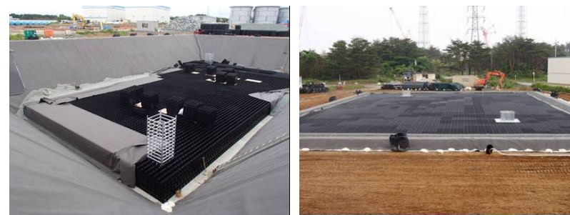
Fig. 2: Installation of underground water storage tank
