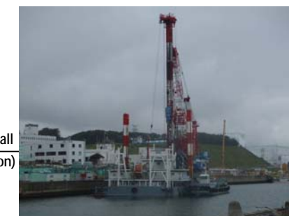
Fig. 4: Preparations of advance boring work for impermeable wall (taken on June 22, 2012)
