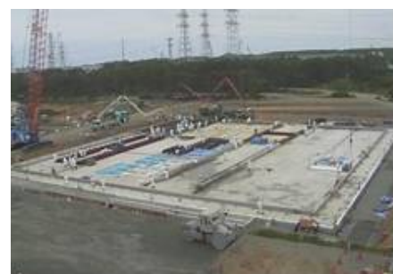
Fig. 1: Foundation work of ALPS
