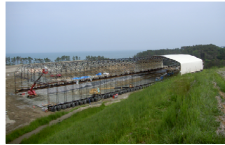
Construction of tent for covering form weather (First facility) [shooting 5/24/2012]
