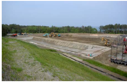
Protective soil work is being carried out (second facility) [shooting 5/24/2012]
