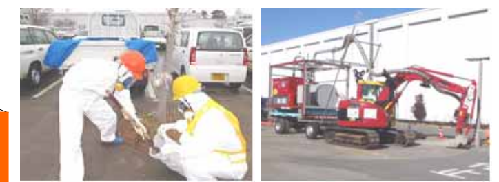
Fig.3 Reducing Dosage Levels in front of the Main Anti-earthquake Building
