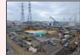
After dismantling in H1 east area
