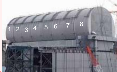
Installation of dome roof (February 21, 2019)
