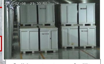
Solid waste storage facility
