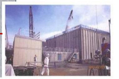
Temporary waste sludge storage
