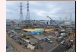
After dismantling in H1 east area
