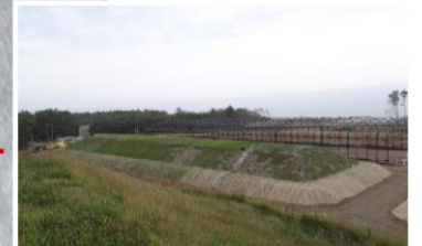
Temporary soil-covered type storage facility
