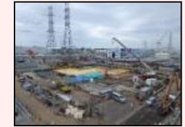
After dismantling in H1 east area
