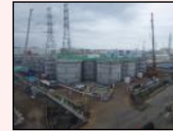
Start of dismantling in H1 east area
