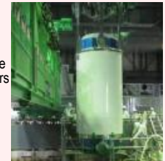
Fuel removal status
