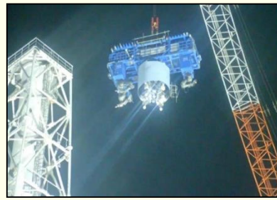
Hanging down of the 3rd block
