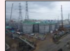
Start of dismantling in H1 east area
