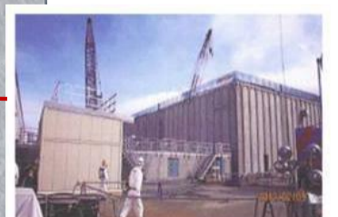
Temporary waste sludge storage
