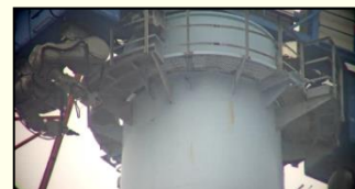
Installation of the dismantling equipment to the stack
