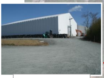
Rubble storage tent
