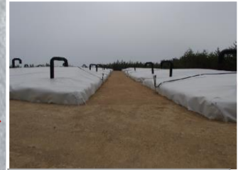
Temporary trimmed trees storage pool
