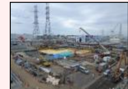
After dismantling in H1 east area
