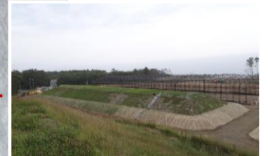
Temporary soil-covered type storage facility
