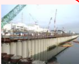
Installation of steel pipe sheet piles for sea-side impermeable wall
