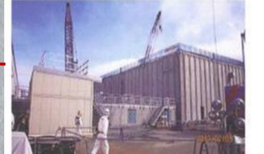
Temporary waste sludge storage
