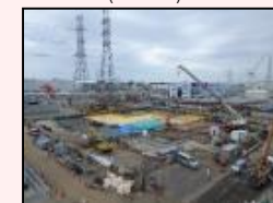
After dismantling in H1 east area
