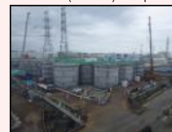
Start of dismantling in H1 east area
