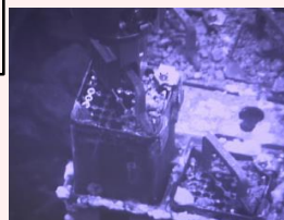
Fuel removal status (April 15, 2019)
