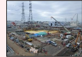
After dismantling in H1 east area
