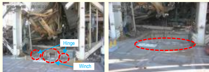
Before removing winches and hinges
