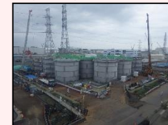
Start of dismantling in H1 east area
