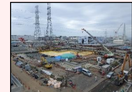
After dismantling in H1 east area
