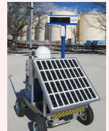
Installation of Dose-rate monitor
