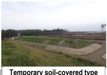
Temporary soil-covered type storage facility
