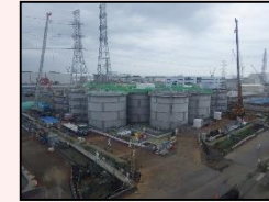
Start of dismantling in H1 east area
