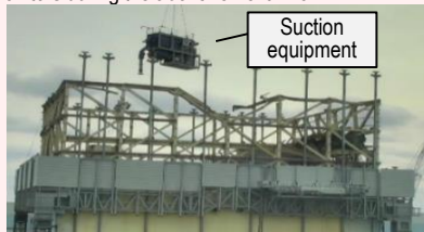
<Installation status (January 22)>
