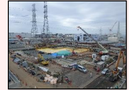
After dismantling in H1 east area
