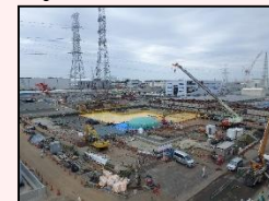
After dismantling in H1 east area
