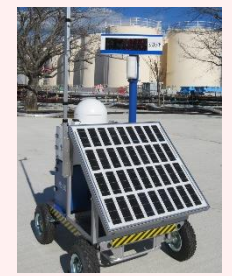
Installation of Dose-rate monitor
