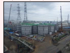
Start of dismantling in H1 east area
