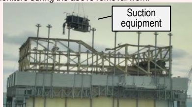
<Installation status (January 22)>
