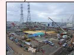
After dismantling in H1 east area
