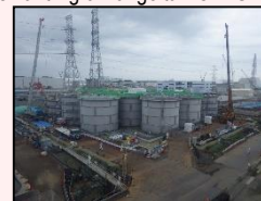
Start of dismantling in H1 east area
