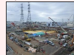
After dismantling in H1 east area
