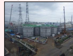
Start of dismantling in H1 east area
