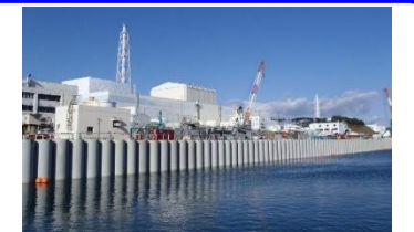
(Sea-side impermeable wall)
