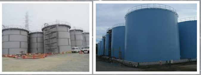
Tank installation status
