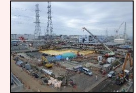
After dismantling in H1 east area
