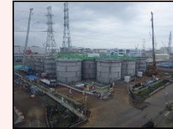
Start of dismantling in H1 east area
