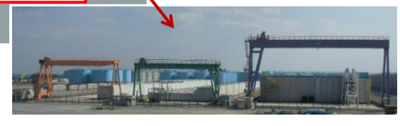
Spent absorption vessel temporary storage
