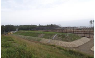
Temporary soil-covered type storage facility
