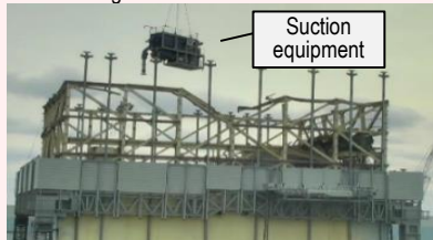
<Installation status (January 22)>
