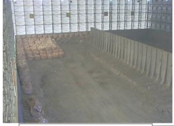
Inside the rubble storage tent
