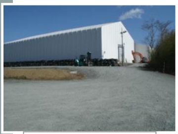
Rubble storage tent
