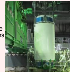
Fuel removal status
