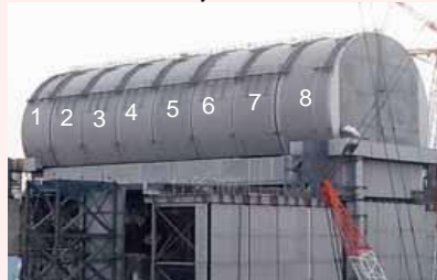
Installation of dome roof (February 21)
