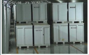
Solid waste storage facility
