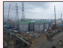
Start of dismantling in H1 east area
