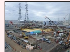
After dismantling in H1 east area
