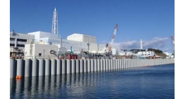
(Sea-side impermeable wall)
