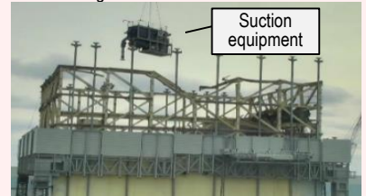
<Installation status (January 22)>
