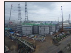
Start of dismantling in H1 east area
