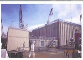
Temporary waste sludge storage
