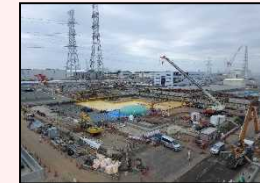
After dismantling in H1 east area
