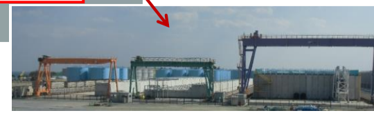
Spent absorption vessel temporary storage
