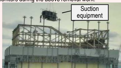
<Installation status (January 22)>
