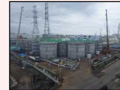
Start of dismantling in H1 east area
