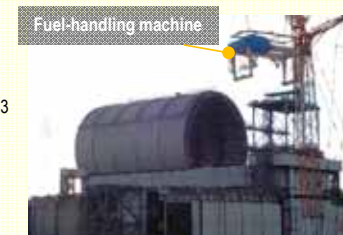
Installation of the fuel-handling machine (November 12, 2017)
