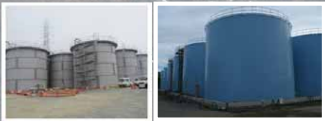
Tank installation status
