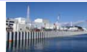
(Sea-side impermeable wall)
