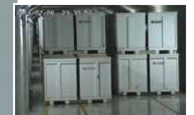
Solid waste storage facility
