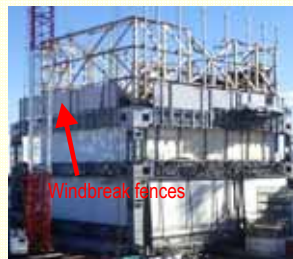
Installation status (November 27, 2017)
