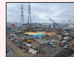
After dismantling in H1 east area
