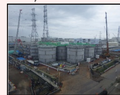
Start of dismantling in H1 east area
