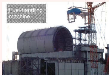
Installation of dome roof (November 12)
