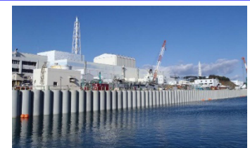
(Sea-side impermeable wall)
