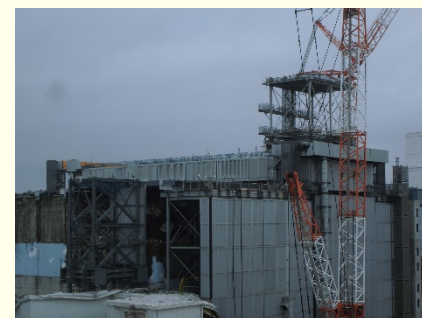
< Installation of the dome roof (installation of slide trestle) >
