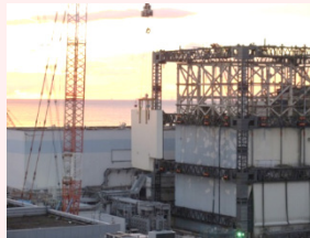
<Dismantling of wall panels>
