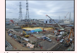
After dismantling in H1 east area
