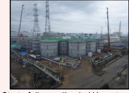
Start of dismantling in H1 east area
