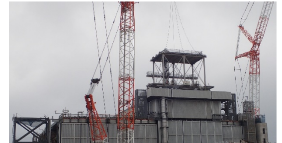
Installation of a cover for fuel removal at Unit 3 (July 26, 2017)
