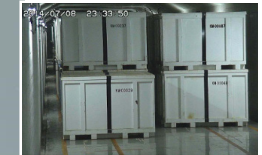
Solid waste storage facility
