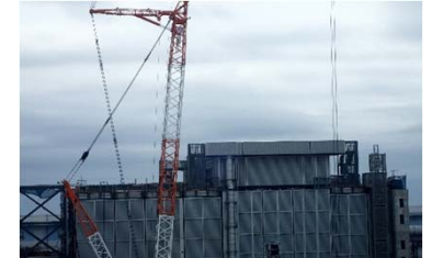
Installation of a cover for fuel removal at Unit 3 (June 27, 2017)
