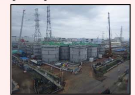
Start of dismantling in H1 east area
