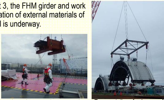
<Lifting of the work floor at Unit 3> <Transportation of a dome roof to the site>
