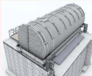
Image of the cover for fuel removal
