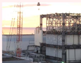
<Dismantling of wall panels>
