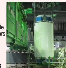
Fuel removal status
