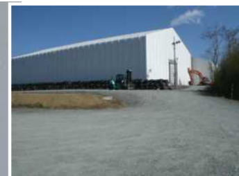
Rubble storage tent
