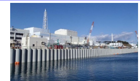
(Sea-side impermeable wall)
