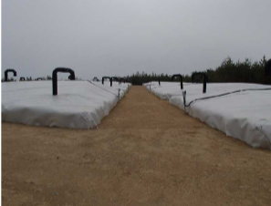
Temporary trimmed trees storage pool
