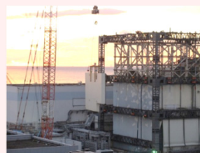
<Dismantling of wall panels>
