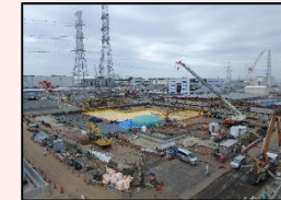
After dismantling in H1 east area
