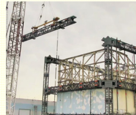
<Removal of beams>
