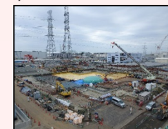
After dismantling in H1 east area
