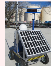
Installation of Dose-rate monitor
