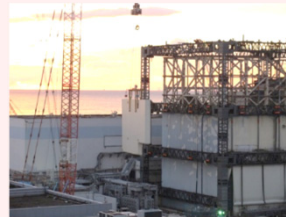
<Dismantling of wall panels>
