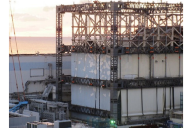
(Dismantling of Unit 1 building cover wall panels)
