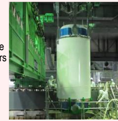
Fuel removal status
