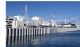
(Sea-side impermeable wall)
