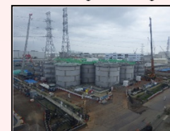
Start of dismantling in H1 east area
