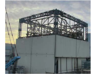
(Dismantling of Unit 1 building cover wall panels)
