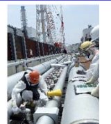
(Opening/closure of frozen pipes)
