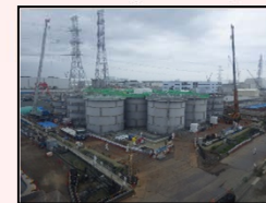
Start of dismantling in H1 east area
