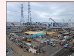
After dismantling in H1 east area
