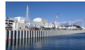
(Sea-side impermeable wall)
