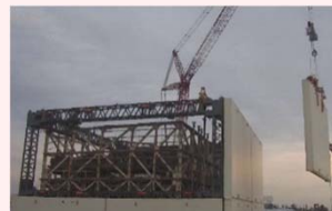
<Dismantling of wall panels>
