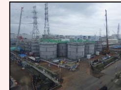
Start of dismantling in H1 east area
