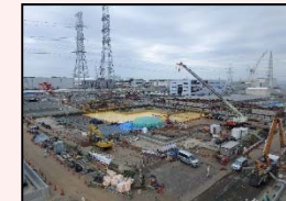
After dismantling in H1 east area
