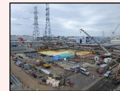
After dismantling in H1 east area
