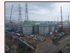
Start of dismantling in H1 east area
