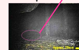
Investigation inside PCV
