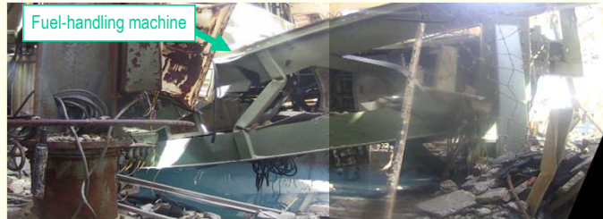
<Investigation of rubble on the Reactor Building top floor (southeast part of FHM)>
