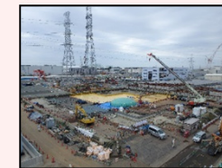
After dismantling in H1 east area
