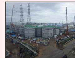
Start of dismantling in H1 east area
