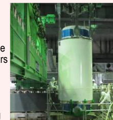
Fuel removal status
