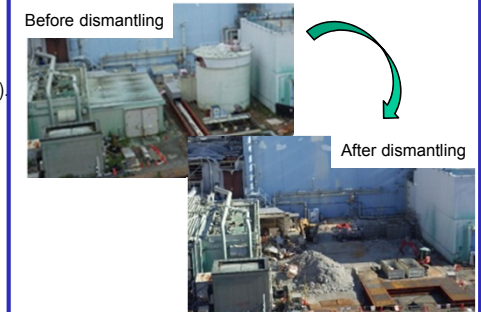
(Preparation around the Unit 2 Reactor Building)
