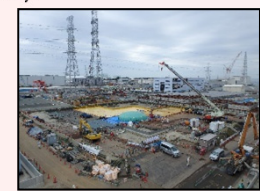
After dismantling in H1 east area
