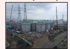
Start of dismantling in H1 east area
