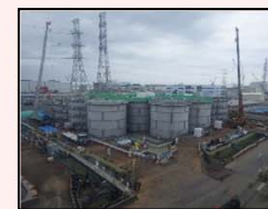
When dismantling started
