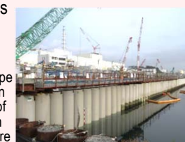
Installation of steel pipe sheet piles for sea-side impermeable wall
