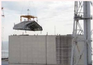
Status of removal of roof panels
