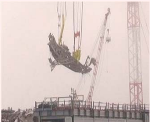
Removal of fuel-handling machine on August 2
