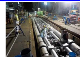
(Installation of pipes for land-side impermeable walls)
