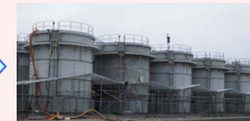
After installing the fence cover
