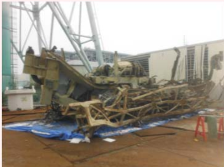
Fuel handling machine removed from the pool
