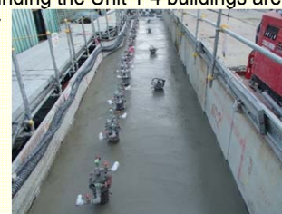
<Sea side of land-side impermeable walls - Installation of frozen pipes>
