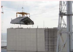
Status of removal of roof panels
