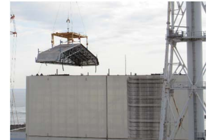
(Dismantling of the Unit 1 building cover)
