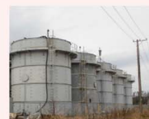
Before installing the fence cover
