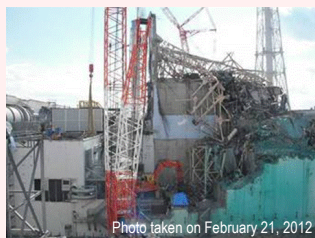
Photo taken on February 21, 2012 Before removal of the large rubble
