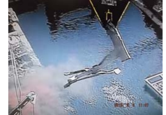
(Mar 6, 2015: Removal of fuel-handling machine west-side frame)
