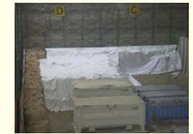
<Status of cover over rubble in tent>
