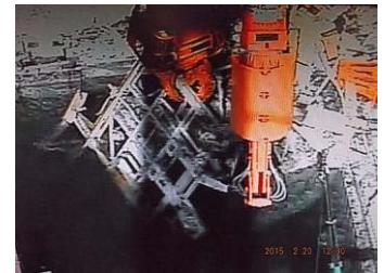
(Feb 20: Removal of fuel-handling machine trolley 2 nd floor)
