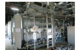
(Land-side impermeable walls freezing plant installation status)
