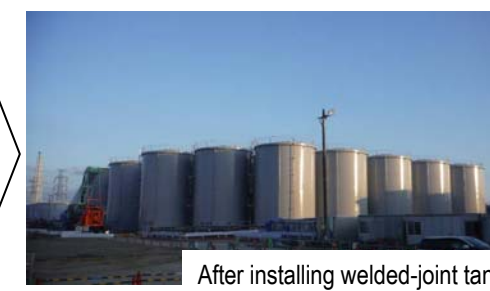
After removing square tanks
