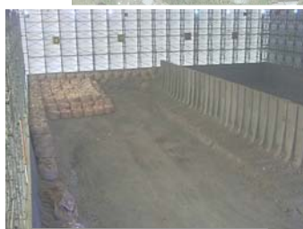
Inside the rubble storage tent
