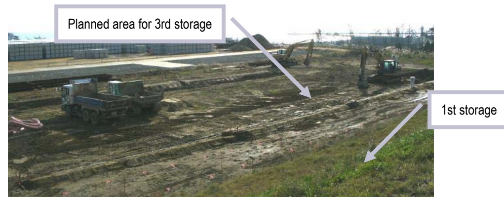
Figure 11: Temporary soil cover-type storage – Drilling status of 3 rd installation area
