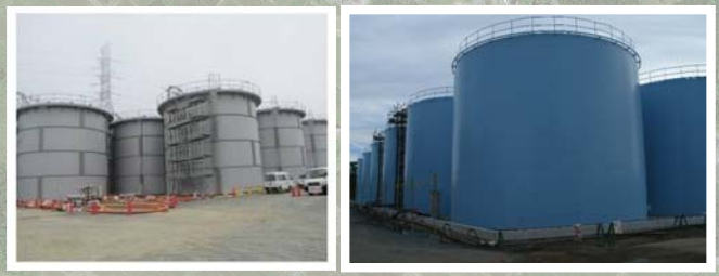
Tank installation status
