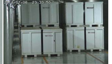
Solid waste storage
