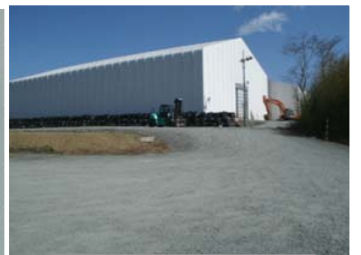
Rubble storage tent
