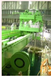
Fuel removal status
