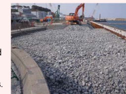
Installation status of impermeable walls on the sea side (Landfill status on the Unit 1 intake side)
