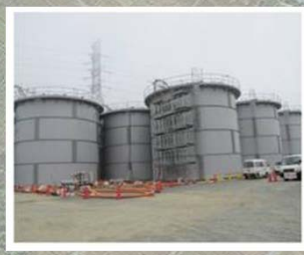
Tank installation status
