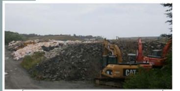
Rubble (outdoor accumulation)
