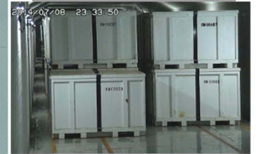
Solid waste storage
