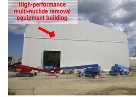
Figure 5: Overview of high-performance multi-nuclide removal equipment
