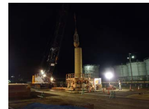
<Status of drilling>
