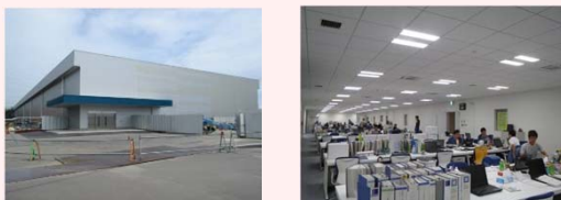
External and internal appearances of the New Administrative Office Building
