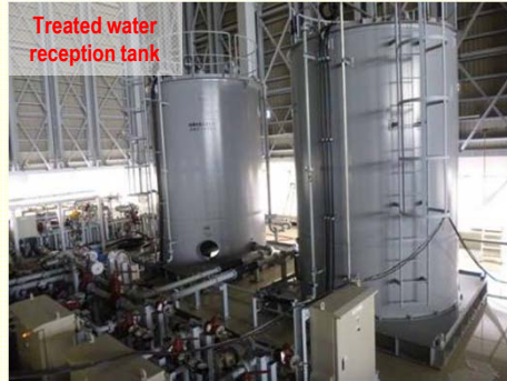
<Installation status of additional multi-nuclide removal equipment>
