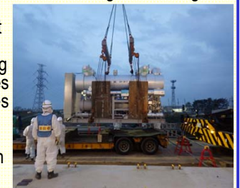
<Installation of chillers for freezing>
